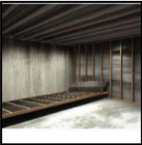
Make sure to leave excess vapor barrier at the corners so that you can wrap it, overlap the seams and tuck tape (not duct tape) them shut. Then fill all holes in studs and joists with fire rated penetration sealant to reduce air movement.
